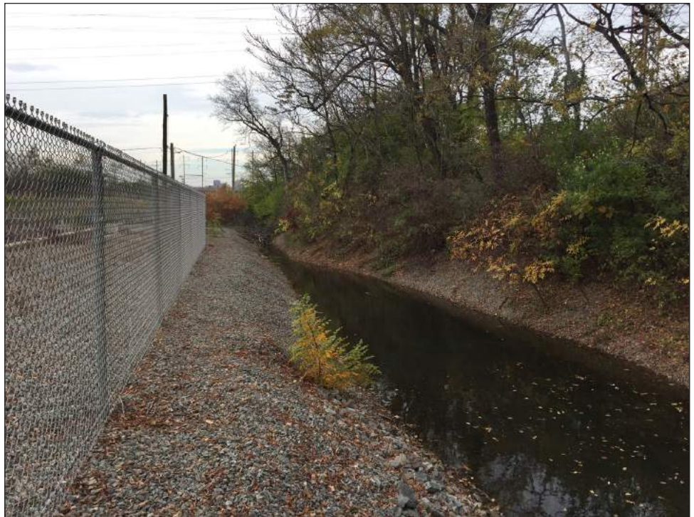
View of Detention Basin E, facing west. 4
